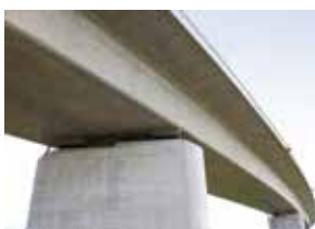
Concrete peeling prevention construction method applicable to wet surfaces
