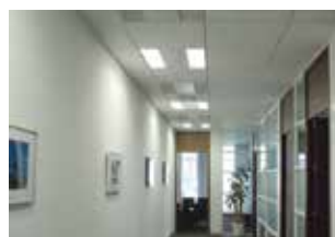
Partial uninstallation of fluorescent lights (Headquarters in Tokyo)
