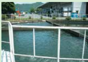
Effluent treatment facility (Shiga factory)
