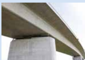
Concrete peeling prevention construction method applicable to wet surfaces
