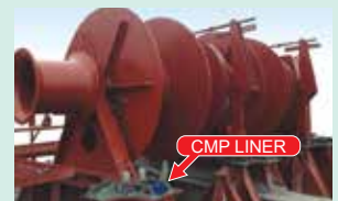
Epoxy resin for chocking CMP LINER
