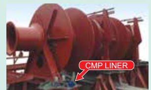
Epoxy resin for chocking CMP LINER
