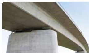
CONTECT WE100 construction method
