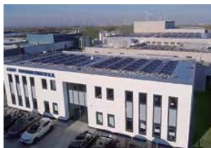
Solar power generation system at our subsidiary in the Netherlands
