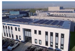
Solar power generation system at our subsidiary in the Netherlands
